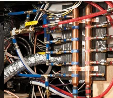
A copper water manifold comes standard, ensuring equal water pressure throughout your home. And each water line is clearly labeled and has its own shut-off valve, allowing you to isolate a single line without shutting off water to the rest of your home.
